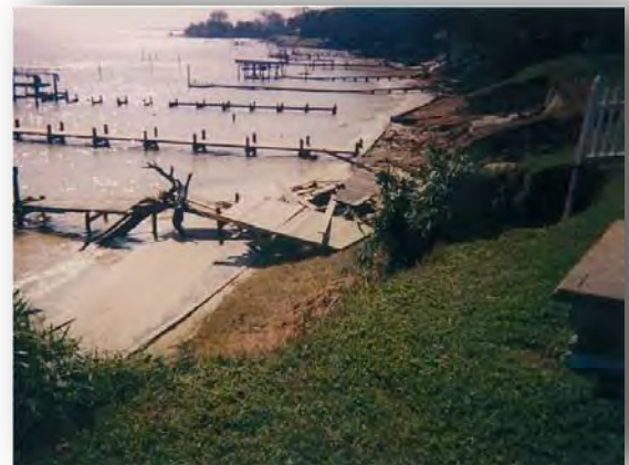
Storm damage incurred on the York River during Hurricane Isabel, 2003. Photo credit: J. Rickards.
